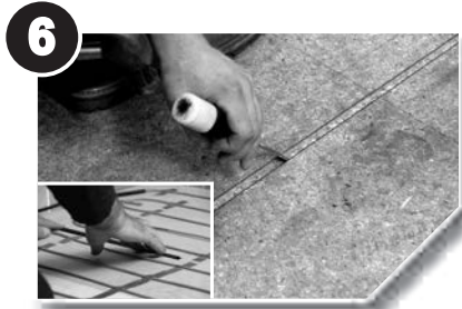
Cut a channel in the subfloor to accommodate the floor probe
