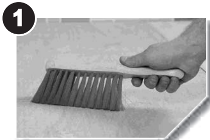
Ensure floor is clean & dust free
