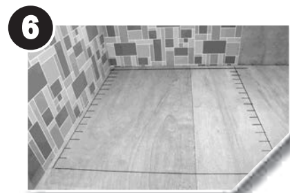
Mark perimeter & cable spacing
